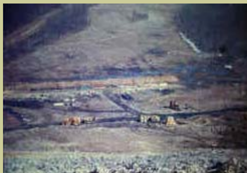
Construction of I-80 in the 1960's near Jonathon Run.
