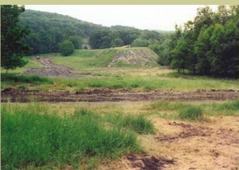
Storage area for fill, and concrete plant.
